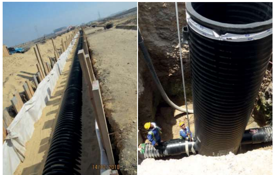
Figure 5: Pipe installation (New Mena Plast, Egypt) and manhole installation (UGPM, Oman)
